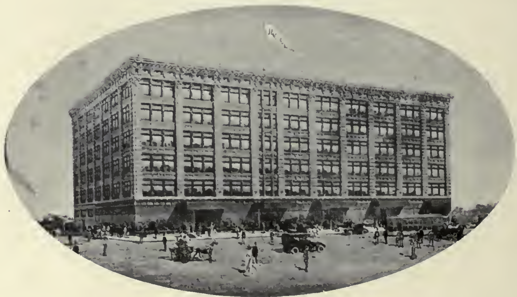
THE JACOBS BUILDING.
